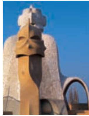
From the flat roof of La Pedrera, where Gaudí transforms the chimneys and ventilation pipes into anthropomorphic sculptures, the Sagrada Família can be seen
