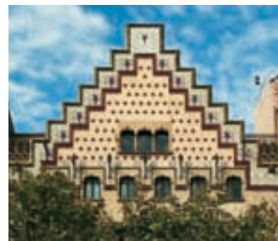
The decoration of the Modernista façades is exuberant, like that of the Casa Amatller, in which the staggered top is highlighted by the application of ceramic elements
