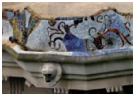
The trencadís technique (composition of broken ceramic elements), reaches the highest possible level of decorative and chromatic expression in the surface treatment of the bench of the Park Güell
